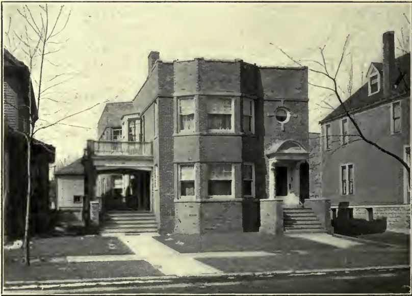
RESIDENCE IN OAK PARK.
